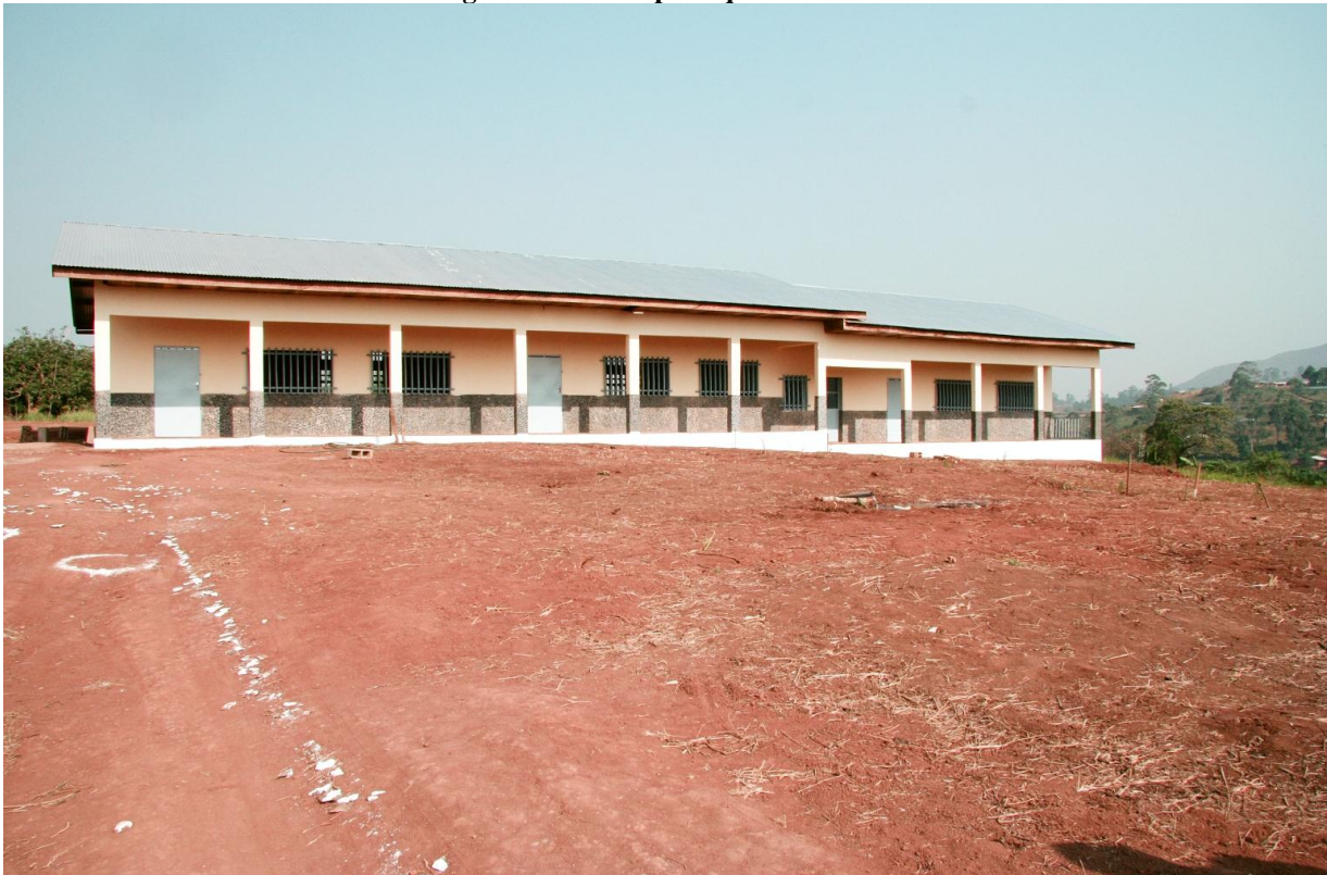
Figure 12 - Ecole publique de Batack
